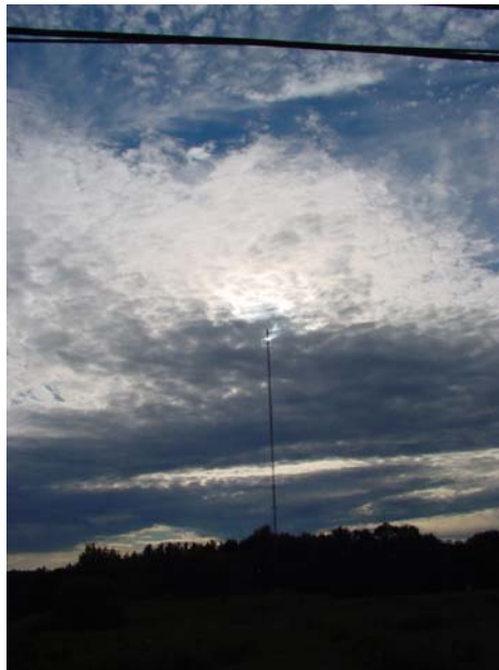
Figure 2: The single tower for radio station WGAW. The tower is a mast tower with a non-directional, circular broadcast pattern (picture courtesy of http://gallery.bostonradio.org/2004-08/worcester/100-02202-med.html )
